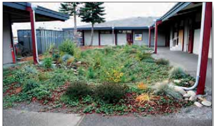
Completed rain garden at Yelm High School
